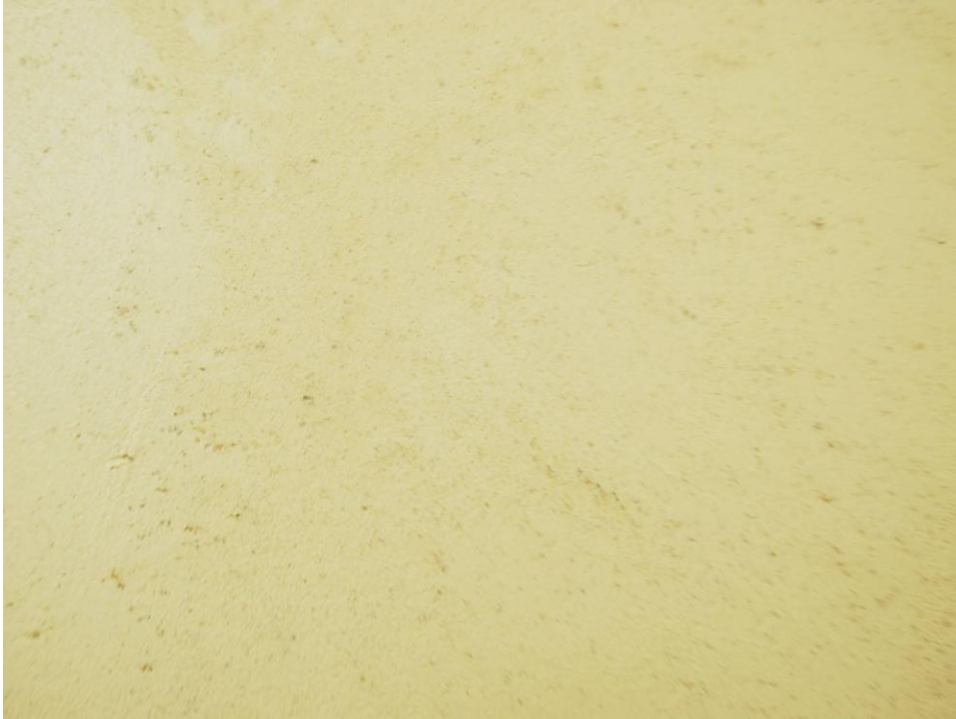
Finished second coat of Tierra™.
