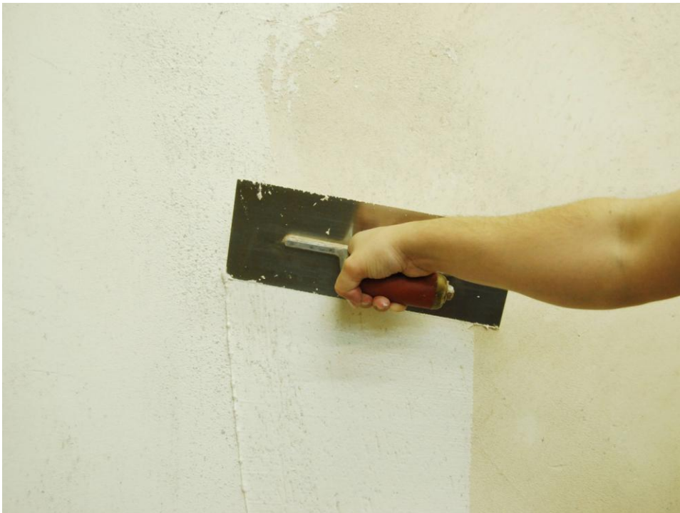
Apply a second coat of Anciano™ using random, decorative trowel strokes.
